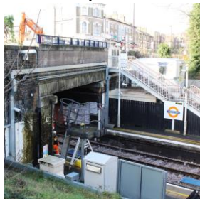
Work has started on preparing Bridge 14 at Crouch Hill for jacking 30cm higher to provide the required clearances for the overhead line equipment. Both 10.01.2018 [KF]
