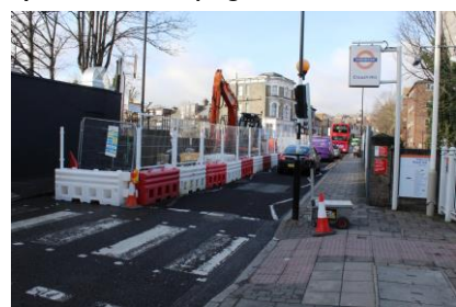
Work has started on preparing Bridge 14 at Crouch Hill for jacking 30cm higher to provide the required clearances for the overhead line equipment. Both 10.01.2018 [KF]
