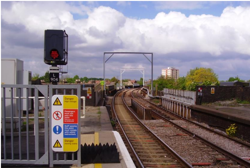
20mph Temporary Speed Restriction at the London end of Wanstead Park, note the way-beam bridges which still remain in this area. [26.04.2017]
