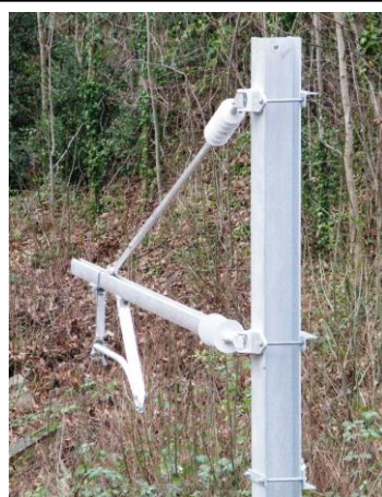
A single line overhead mast near Crouch Hill, note registration arm tied up with blue string! 2 nd February 2017.
