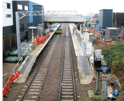
Lift towers under construction at Blackhorse Road station on 6 th January 2017.
